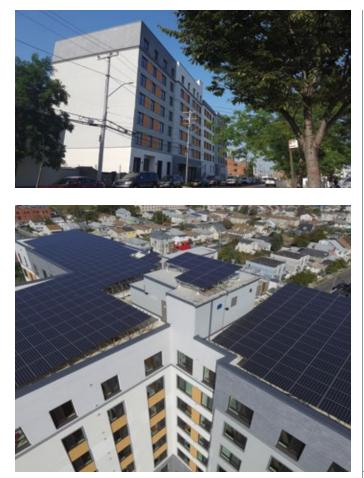
A 133 kWh solar array on the roof supplies nearly all of building's energy needs.
